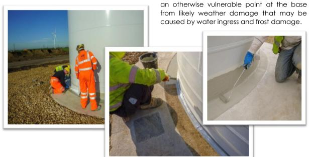
**The outcome:** The completed repairs provided reinforced waterproofing around the bases of the wind turbines along with a warrantee for the high quality waterproofing system, resulting in
